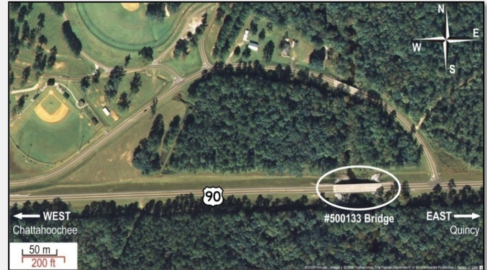
Localization of the tested bridge
