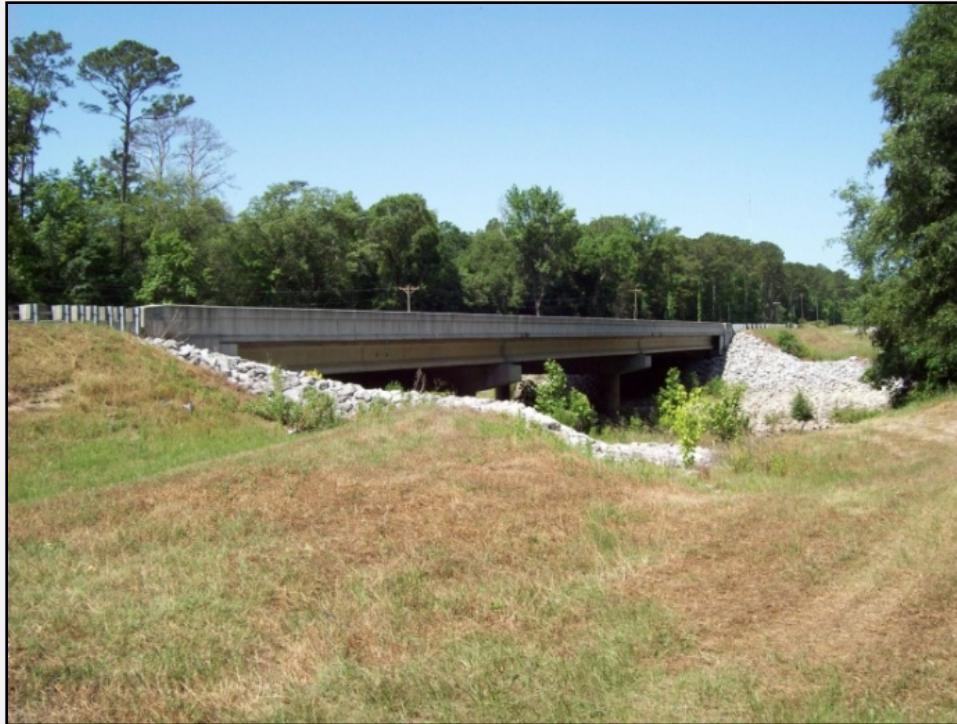
The bridge #500133 over Mosquito Creek
